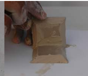
Apply the slip and fix the square slab
